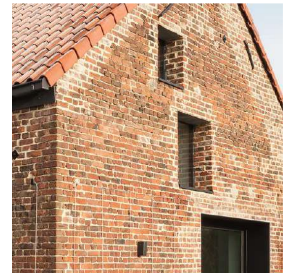
IRREGULARLY ARRANGED FENESTRATIONS
