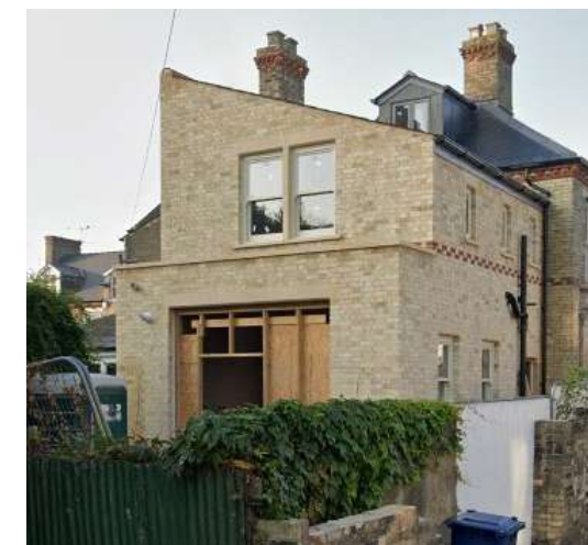
58 CARLYLE RD, EXTENSION IN THE CONSERVATION AREA
